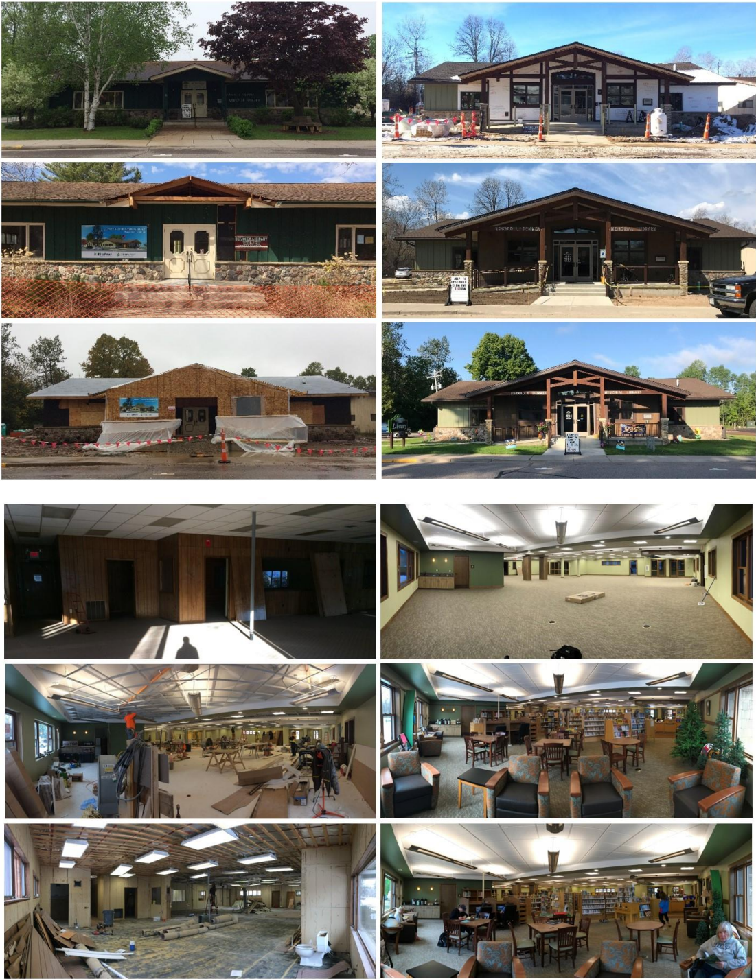
Features of remodeled building: LED lighting throughout, high efficiency furnaces and HVAC upgrades including zoned programmable thermostats, rainwater retention ponds for stormwater runoff management – landscaping to be completed with natives and pollinator-friendly species. All aspects of the public space are considered “educational” in nature; collections include special collections curated by the Three Lakes Waterfront Association ( http://tlwa.org/ ) and those supporting Three Lakes as a Bird City.
